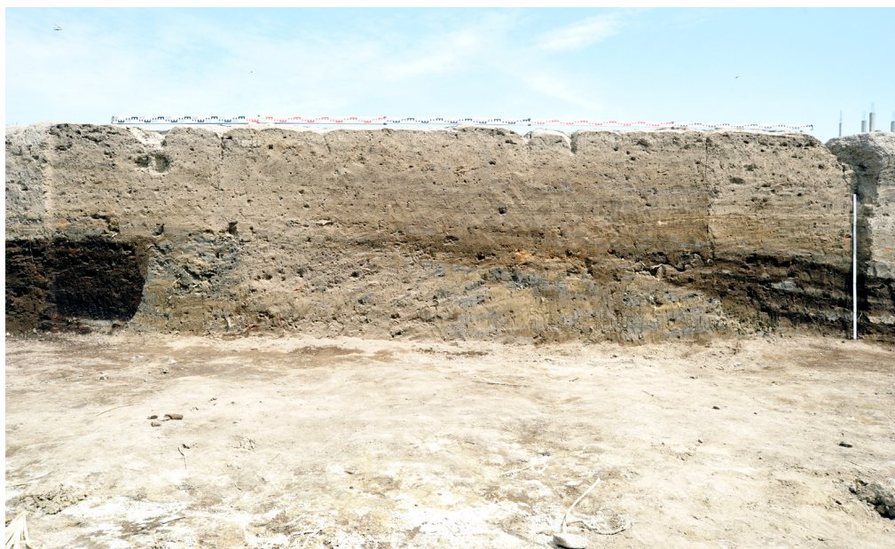
9. Destroyed room and the burnt layer extending north and south of it; view from the west (Phot. R. Słaboński).
