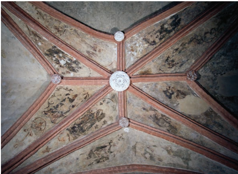
Fig. 5. Starry vault with uncovered murals, the condition after maintenance works, June 2017, photographed by J. Raczkowski.
