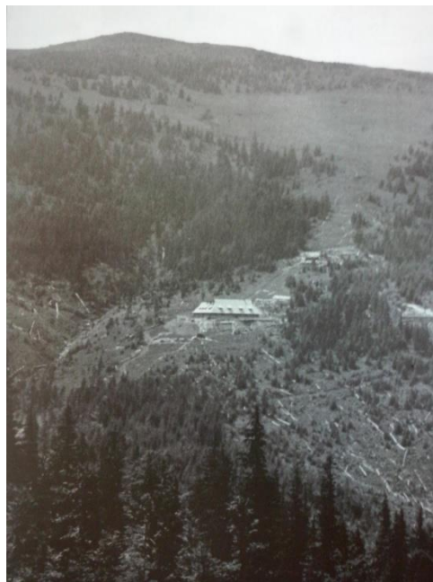
Fig. 2. Shelter at the foot of Kukul mountain
