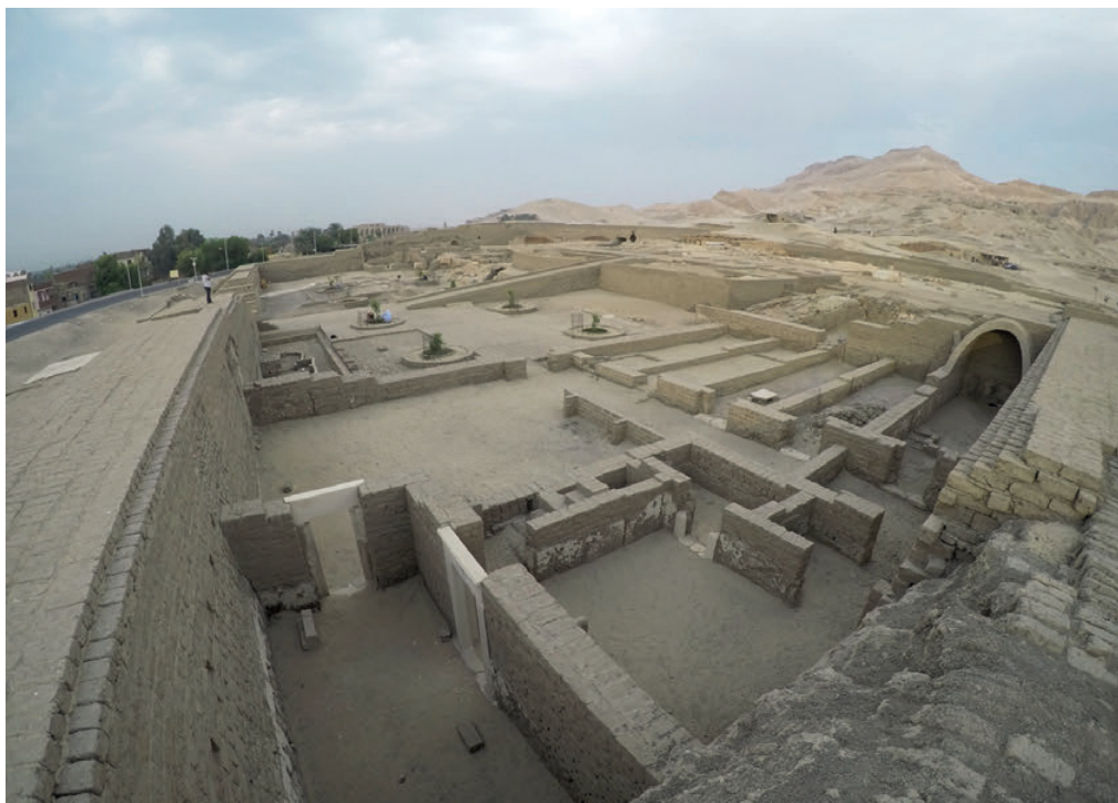
11. Mudbricks buildings to the North of the second courtyard (Phot. I. García Martínez © Thutmose III Temple Project).
