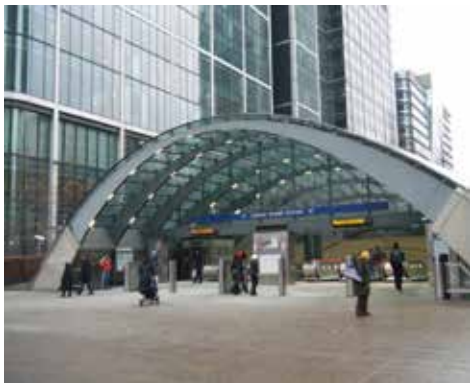
Photo 11. Jubilee line station
