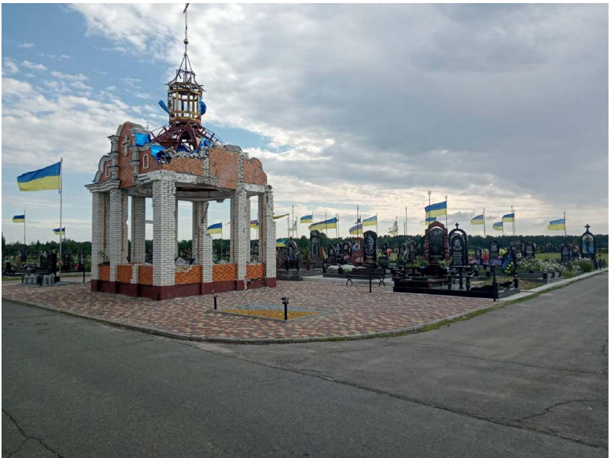
Figure 2. Evidence of structural damage to the memorial infrastructure at “Yatsevo” cemetery resulting from shelling in February – March 2022. The ruins of the memorial chapel near the ATO participants’ burial sector (June 2022)
