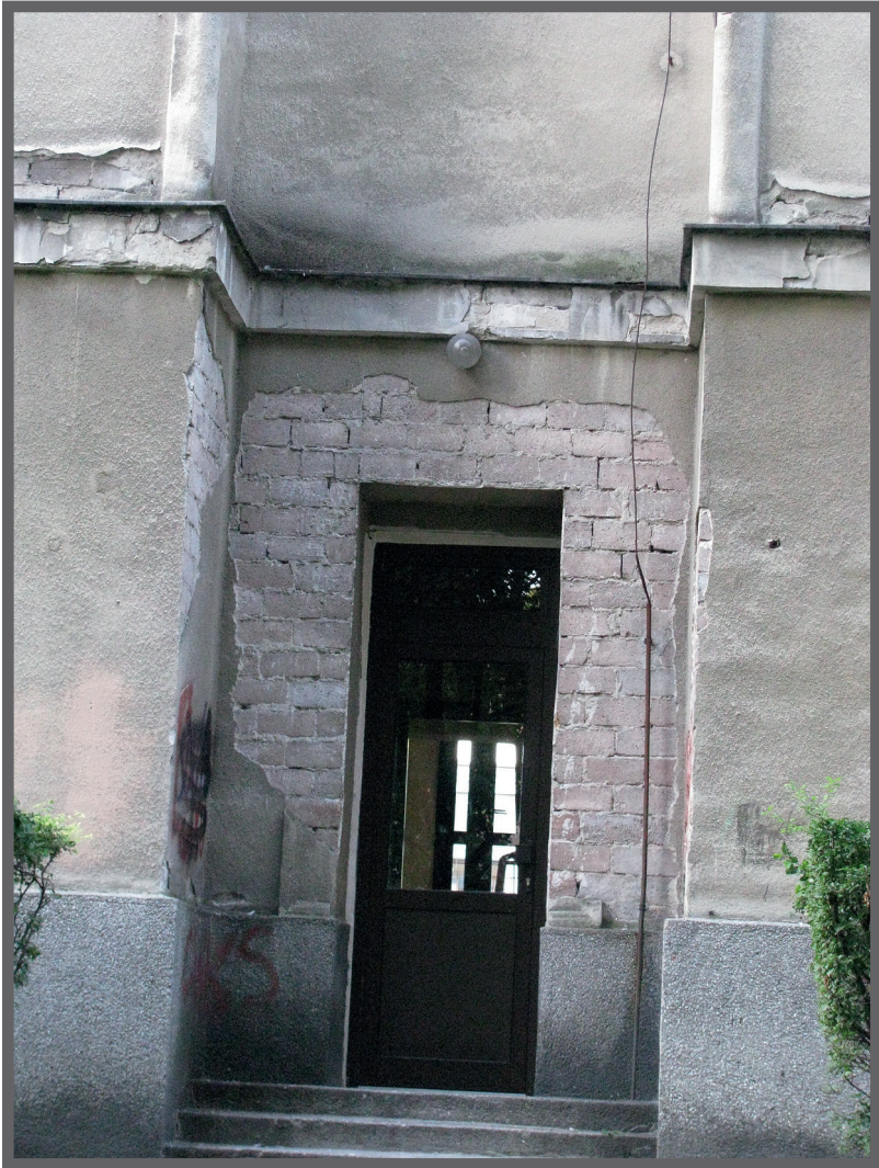
Ill. 7. Muranów housing estate – building with uncovered parts exposing rubble elements, ph. Paulina Świątek (2011)
