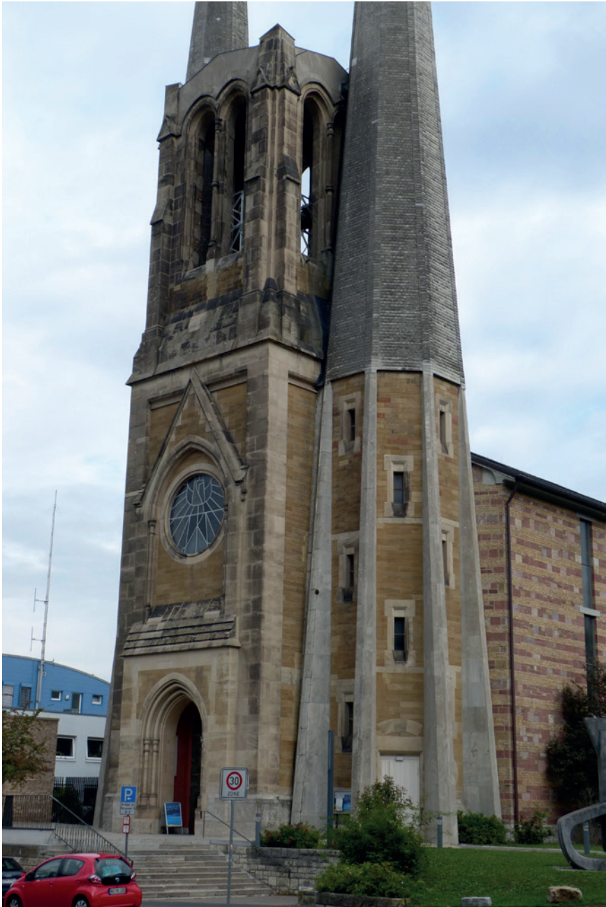
Fig. 7: The front elevation of St. John's Church with the former neo-style tower. Photo. Kazimierz S. Ożóg
