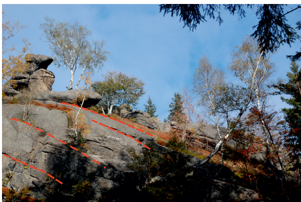
Fig 5. Sheeting joints (red dashed lines) and the convex rock slope in the half dome at Starościńskie Skały
