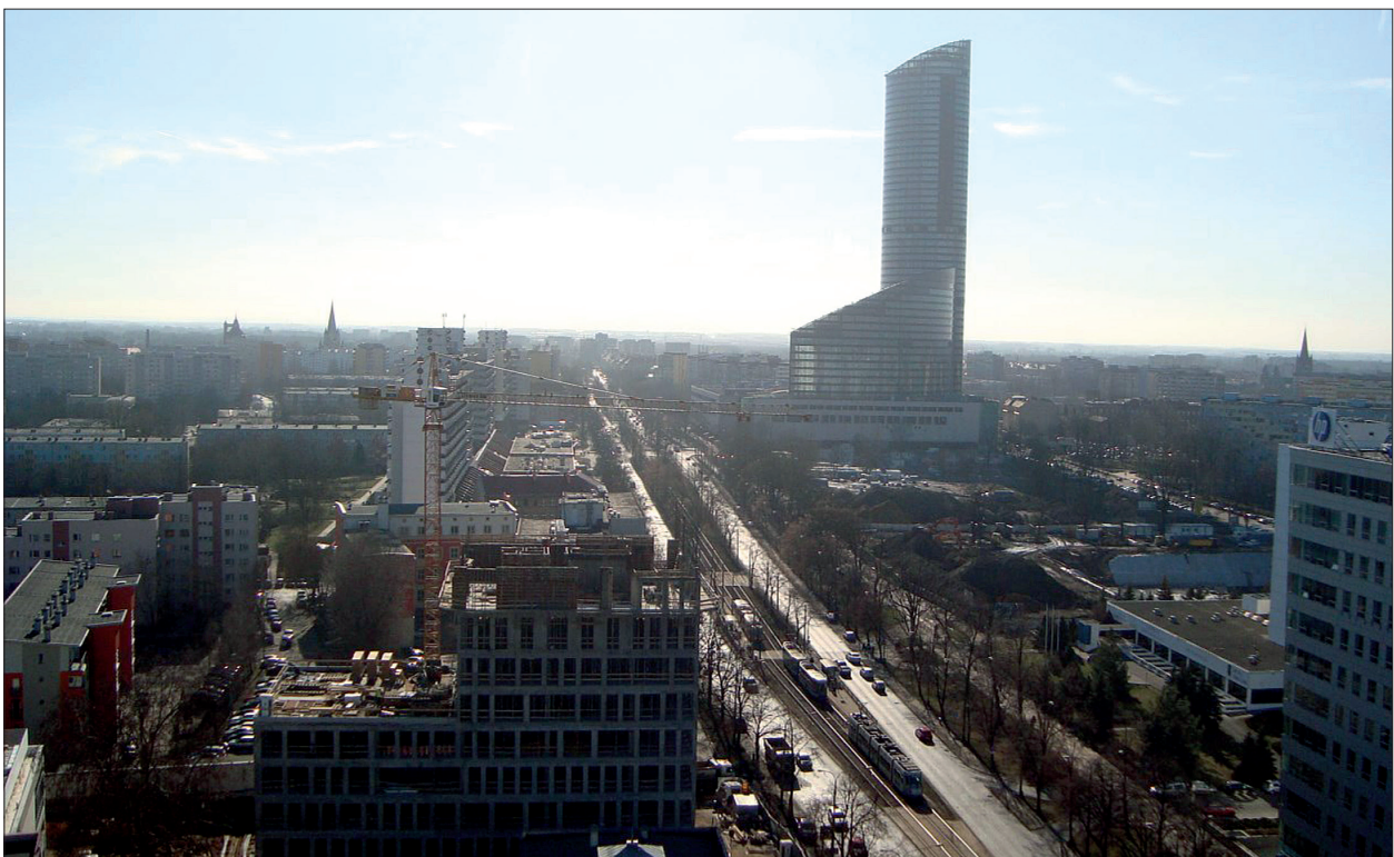
Fig. 13. The Sky Tower in Wrocław city, the view from the north
