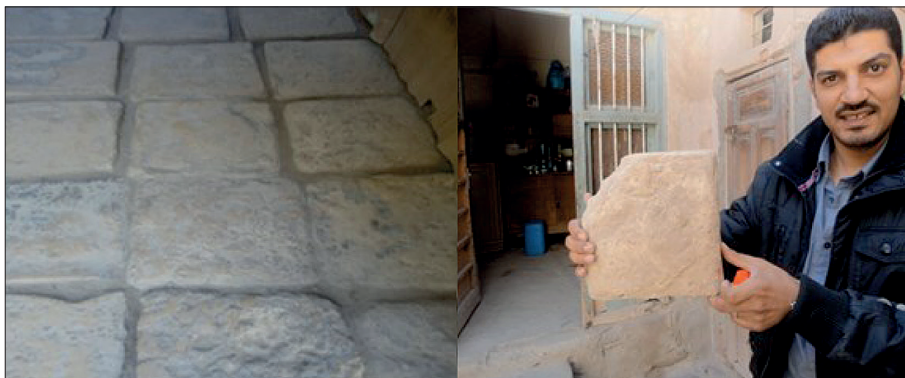
Fig. 8. Farshi Bricks Used in Flooring Courtyards of the First Phase Houses
