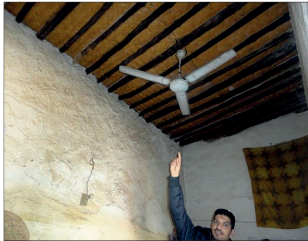
Fig. 6. A ceiling constructed with wood and mud at one of the houses of the old city
