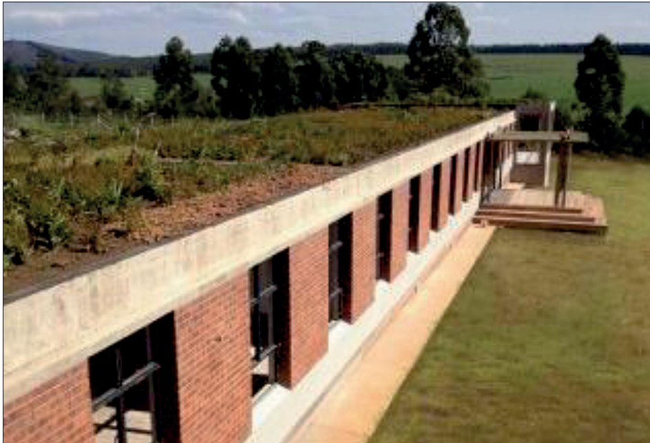
Photo 1. A four star rated government building
