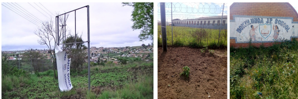
Fig. 9. School closure (left) and deteriorating school infrastructure (right)
