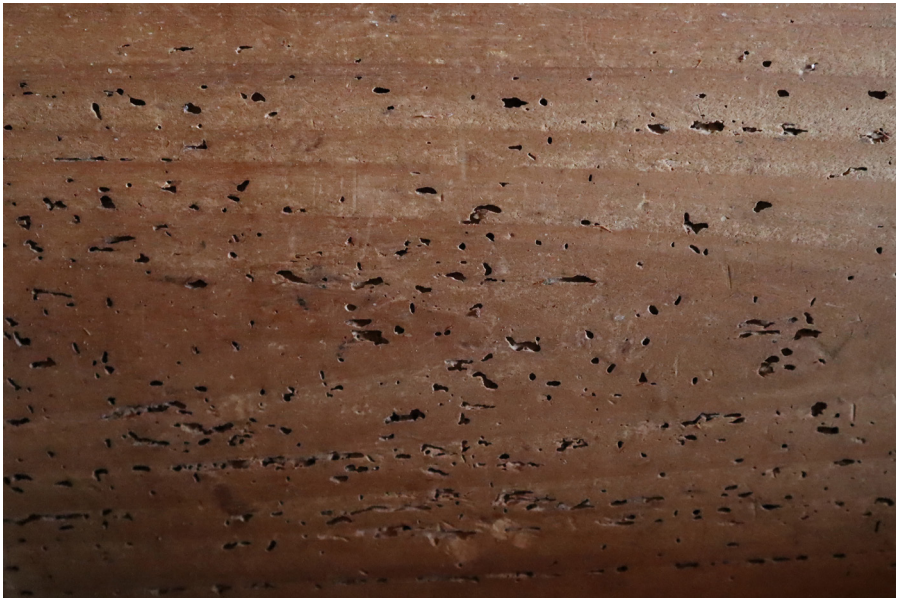
Fig. 3. Inner wall of the cassone no. 1 (ΞΛ23). Tangential section with traces of wood boring insects. Photo: the authors
