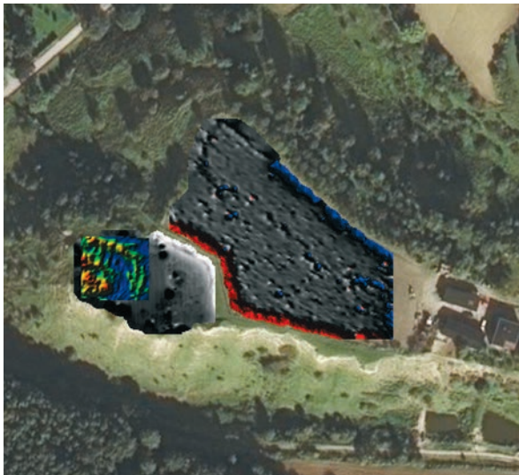
Fig. 7. Unisław, Chełmno district. Altitude plan of the castle with its outer baileys (edited by P. Molewski)
