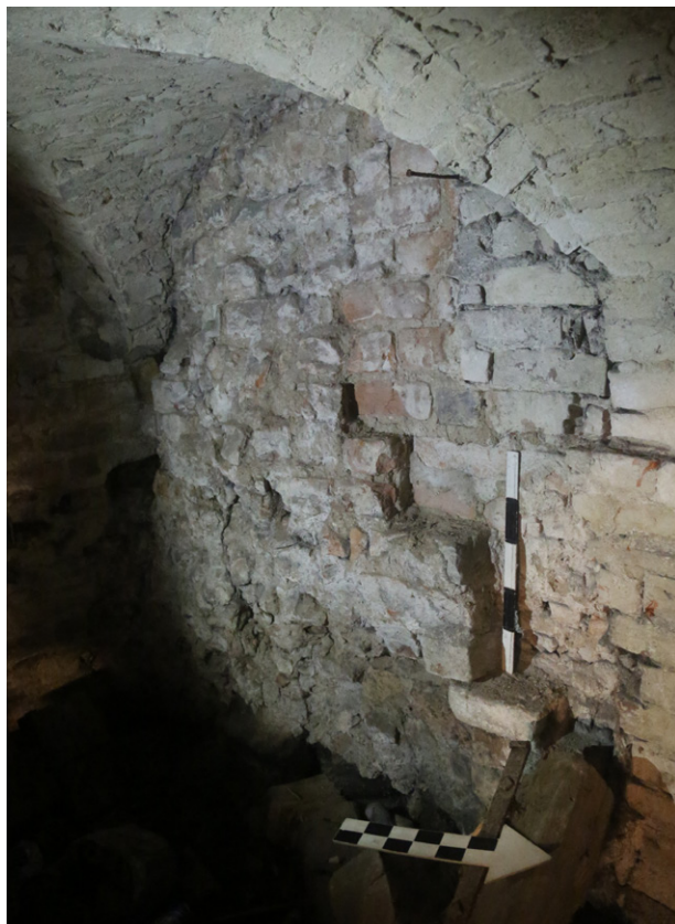
Fig. 8. Toothings visible in the crypt at the former junction of the nave and the southern wall of the first chancel of Saint Matthias Church (photo by R. Biel)
