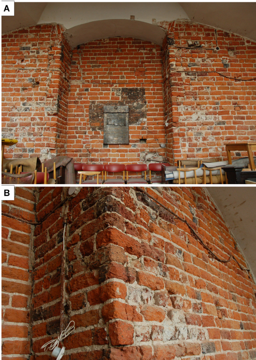
Fig. 6. Western wall of Saint Matthias Church. A – niche interpreted as the base for a planned westwork tower, with visible brick toothings for the intended side walls; B – close-up of the northern tothing, showing traces of medieval reworking and refacing (photo by R. Mruczek; archives of Akme)
