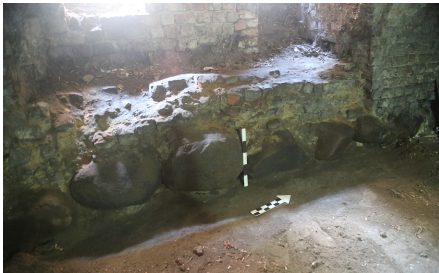
Fig. 5. The niche for the planned westwork tower starts almost at the foundation level, composed of large glacial erratics. In this area, no lower stone layer attributed to the residential tower was identified – only a humus layer was present (photo by R. Biel)
