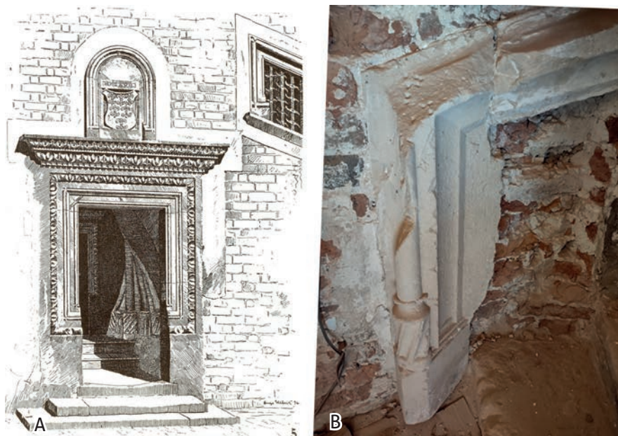
Fig. 7. Wrocław, pieces of masonry included in the southern staircase tower in the years 1518–1527. A – portal in H. Lutsch's drawings, B – the unearthed railing of the spiral staircase prior to the conservation work (photo by M. Chorowska)
