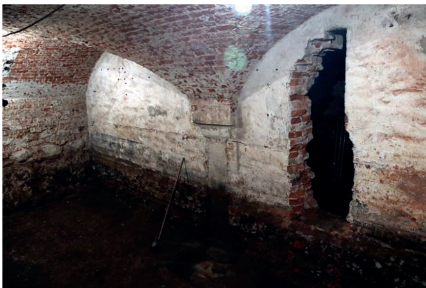
Fig. 2. Wrocław, interior of Piwnica Świdnicka in the underground of the House of the Cathedral Chapter. In the centre of the wall that serves as a secondary partition in the cellar there is a walled-in pillar (photo by M. Bogdała)
