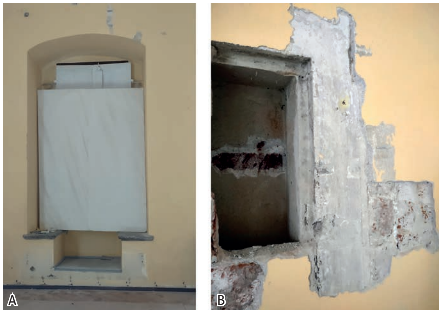
Fig. 6. Wrocław, House of the Cathedral Chapter, window openings on the first floor level: A – recess of the walled-in window opening with stone sedilia on the sides – north, B – walled-in entrance to the north (sanitary?) unit, prior to the conservation work (photo by M. Chorowska)
