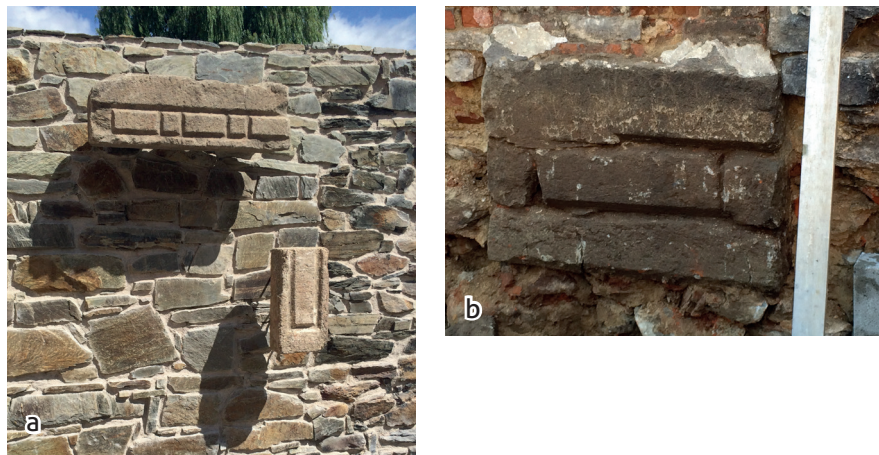
Fig. 5. Głucholaży, the alderman's seat, details of the Renaissance décor: a – elements of the stone framing – probably from the northern wing (currently exposed on the wall), b – the lower part of the pillar of the arcade made of reused Gothic stone framing (photo by A. Legendziewicz)
