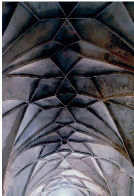
Fig. 3. Brzeg, Friar Minor Church. Vault of the nave, state from 2002 (photo by A. Legendziewicz)
