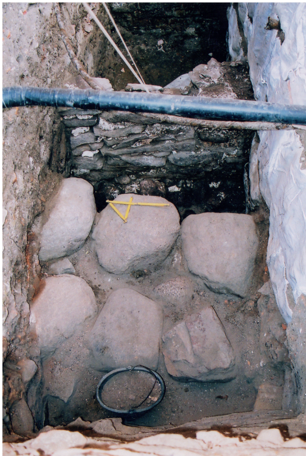
Fig. 3. Continuous foundation on the west side of the church – trench 54 (photo by A. Sikorski)
