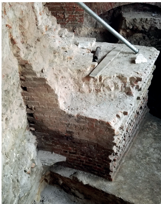
Fig. 9. Wrocław. Arched wall: view from the north. Remains of concave toothing visible on the left (photo by P. Kmiecik)
