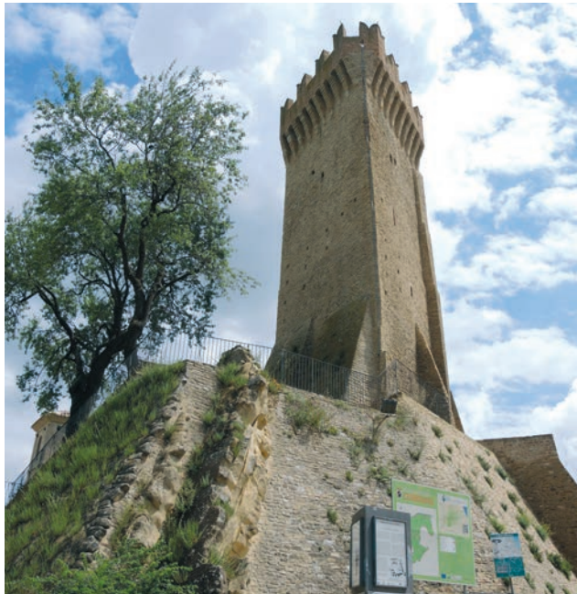
Fig. 4. The triangular tower of Montegualtieri in Abruzzo (after https://commons.wikimedia.org/wiki/File:Torre_di_Montegualtieri_01.jpg )
