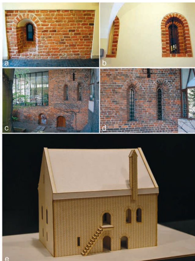
Fig. 9. Wrocław, Old Town. Bourgeois tenement houses from the 13 th century: a – tenement house at Rynek 6; window II. of the storey at the rear of the northern house (13 th century), exposed in the vestibule of a contemporary tenement house; b – windows III. of the storey of the rear wing in the southern house (13 th century), visible in the entrance hall of a contemporary tenement house; c – the so-called Dom Panien Trzebnickich (Trzebnickie Maidens House) at 8 Biskupa Nankera Place; western elevation; d – close-up of the first floor window openings (2 nd quarter of the 13 th century); e – 3D model; student work (photo by R. Mruczek)
